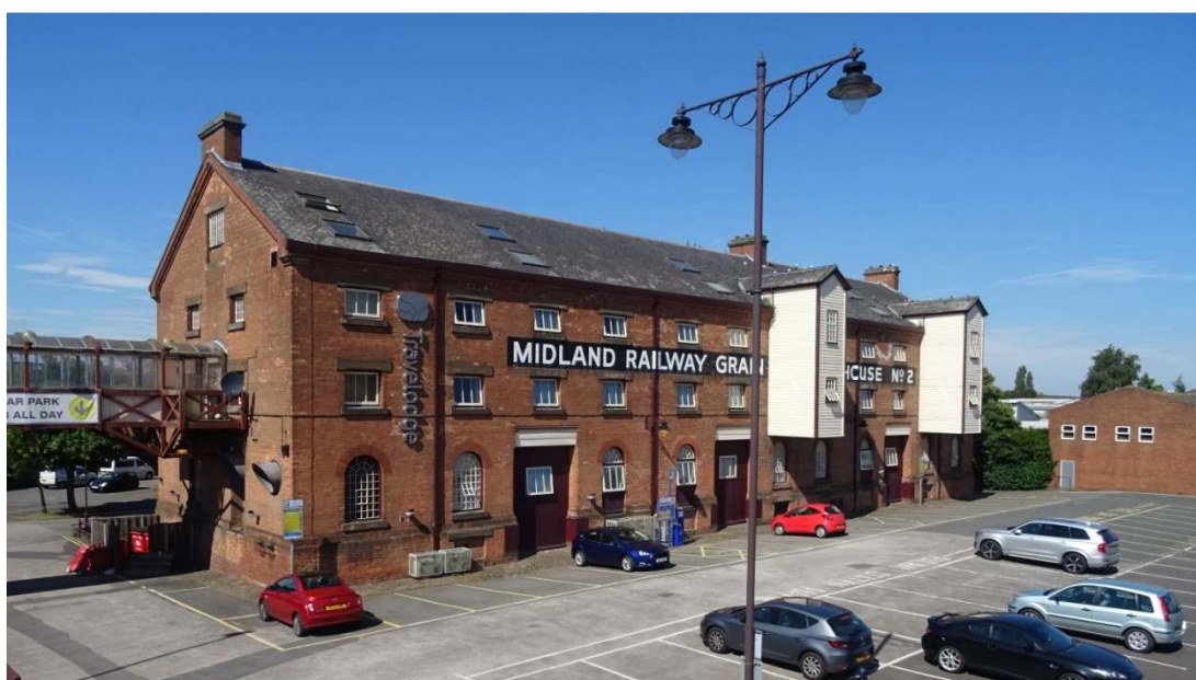
Plate 30: Midland Railway grain warehouse at Burton, now a hotel (asset 1554)
