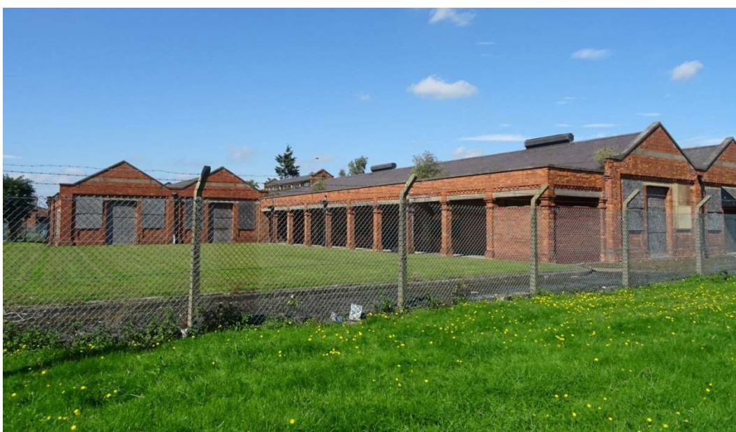
Plate 32: Grade II listed canteen buildings at the WWI machine gun factory (asset 1460)
