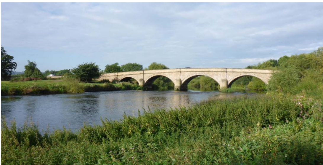
Plate 24: Swarkestone medieval bridge (asset 2888)
