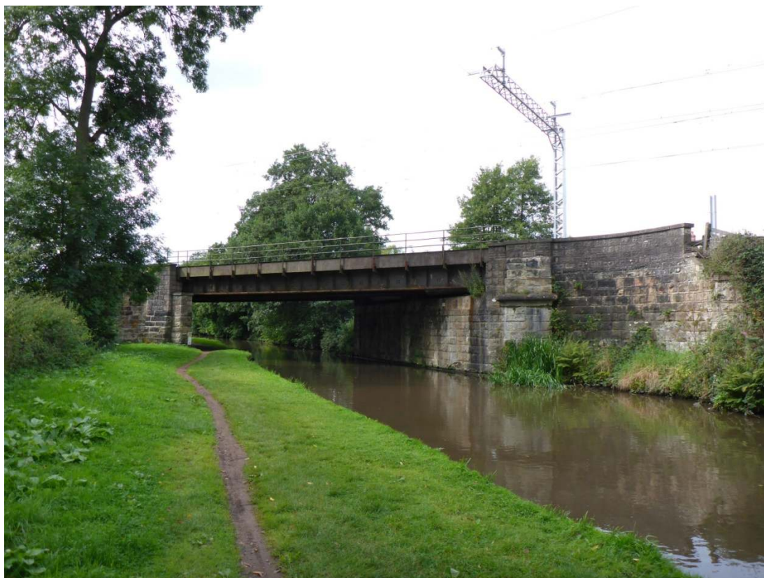
Plate 22: London & North Western Railway bridge over the Trent & Mersey canal at Colwich
