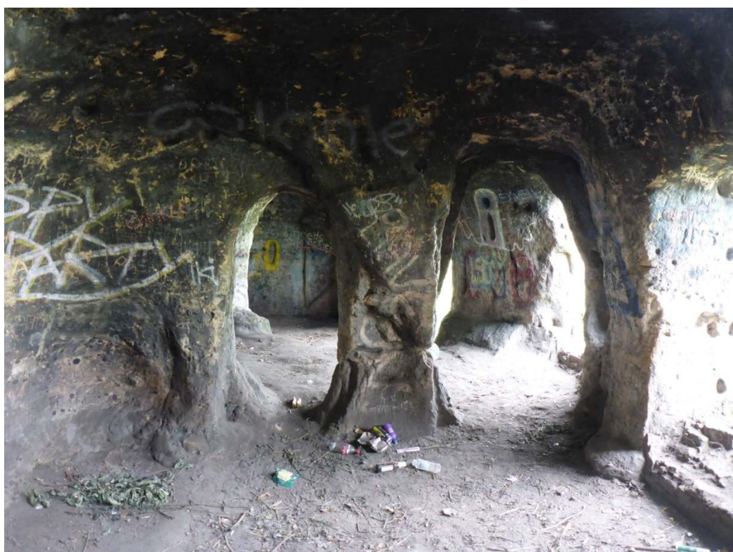
Plate 29: Graffiti, rubbish and smoke damage within Anchor Chapel
